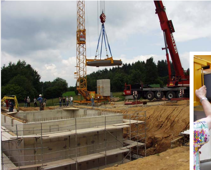
Installation of the Zerodur base plate
