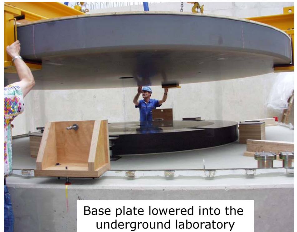
Installation of the Zerodur base plate
